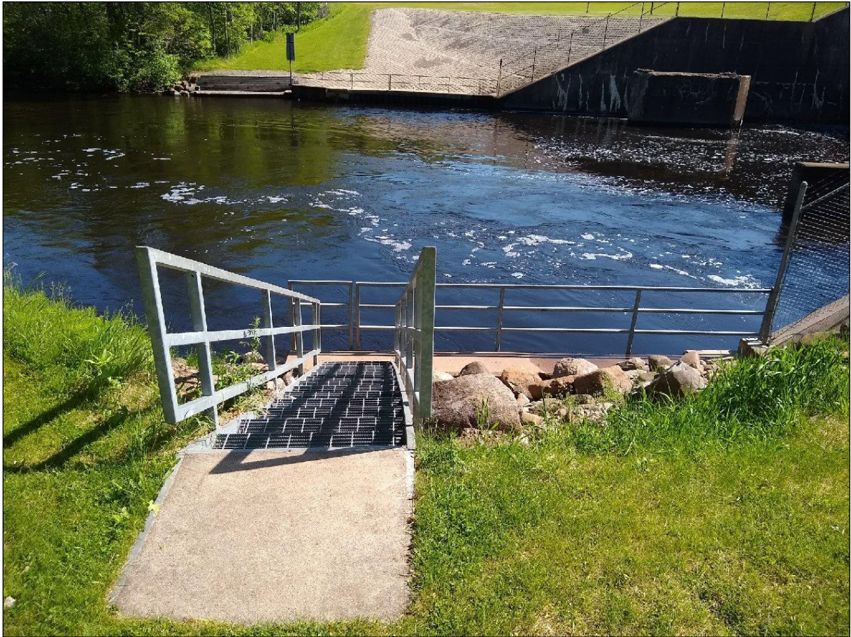
Figure 4.8.2.6-1: South Tailwater Access Stairway and Fishing Platform
