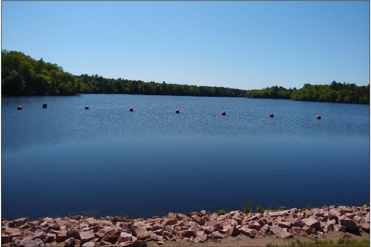
Figure 4.9.1.2-2: View of the Reservoir Upstream of the Trego Dam
