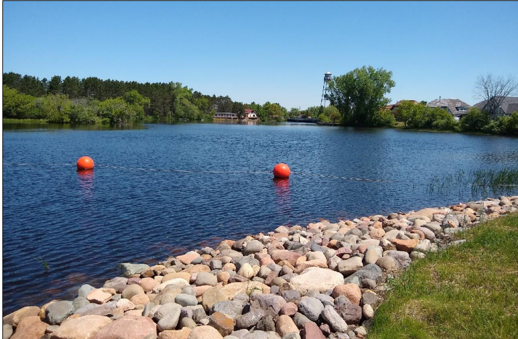
Figure 4.9.1.1-2: View Upstream of the Hayward Dam
