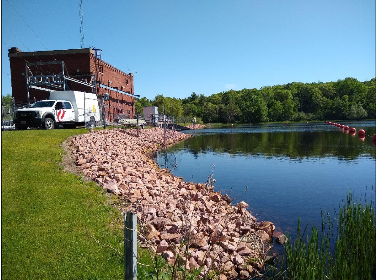
Figure 4.9.1.2-1: View of the Trego Dam
