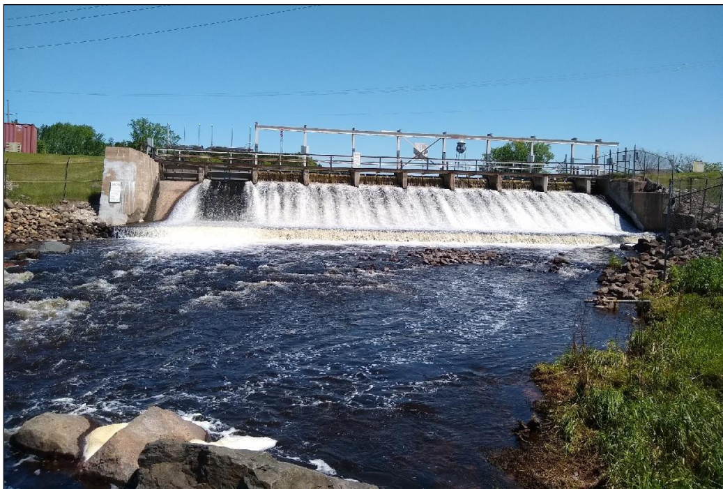
Figure 4.9.1.1-3: Hayward Project Spillway
